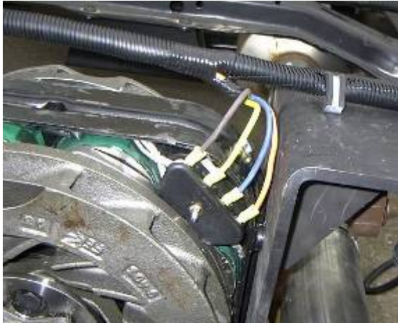
POWER CONNECTIONS AT TOP RIGHT REAR
